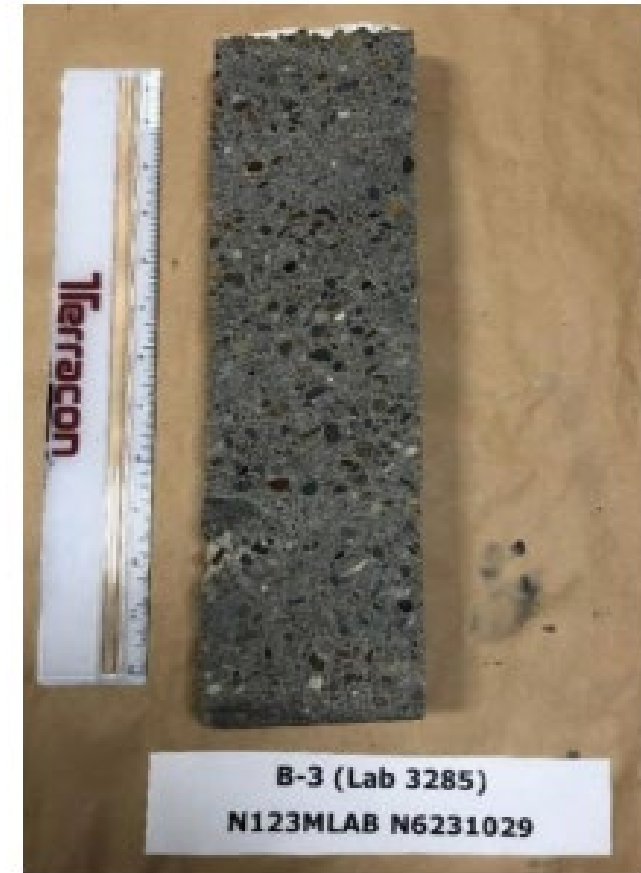
Photo 15: Core B-3 sawn and polished surface. Poor aggregate distribution and evident segregation is noted.
